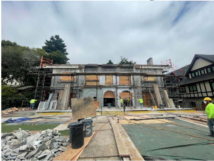
Exterior work on the Delta Delta Lodge at Cal
